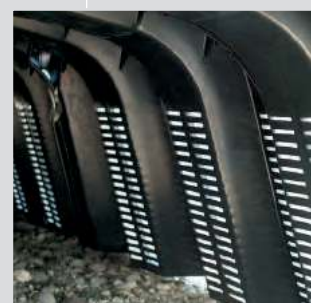
⑤ The base is completely open and side walls are slotted, creating an infiltration surface of 12.400 cm 2 per element.
