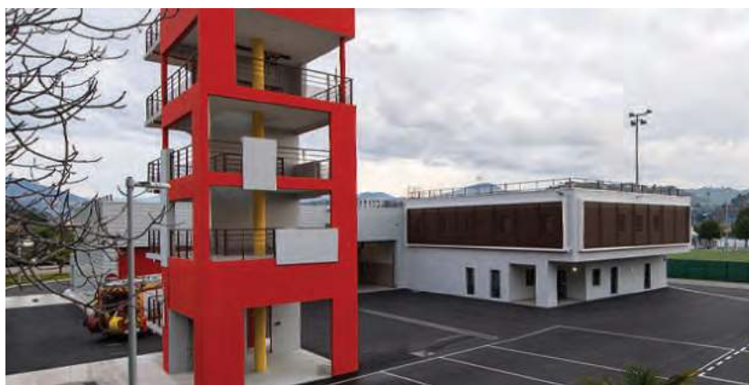
ELEVATOR TANK Firefighting center SAINT-LAURENT-DU-VAR, FRANCE
