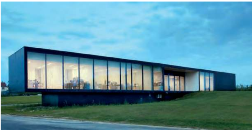
DRENING Marchesini Group HQ PARIS, FRANCE
