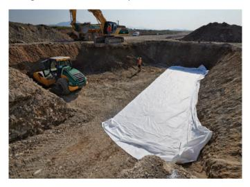
In order to install the AQUABOX and AQUABOX CUBE modules, a flat and stable laying bed is essential. For this aim it is necessary to create a levelling layer of minimum 10 cm above the bottom of the excavation, preferably made of crushed stone or gravel (without fine fractions). The layer must be carefully compacted and smoothed to obtain a flat surface.
