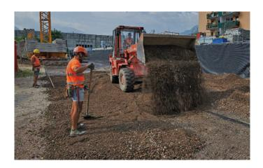
Compression level Dpr must be  $\geq$  97% (Evd  $\geq$  25 MN / m2 or CBR  $\geq$  8% top edge of bedding). If soil has been included in the infiltration calculation, the permeability of the compacted layer must at least correspond to the permeability (kf value) of the backfill soil (soil groups GE, GW, SE, SW, SI).
