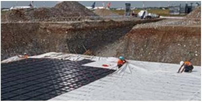
Stormwater infiltration basin (800 m³)
