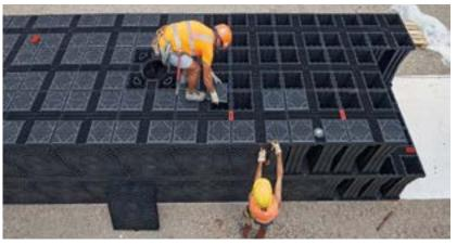
Stormwater infiltration tank (130 m³)
