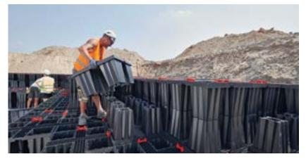
Stormwater infiltration basin (800 m³)
